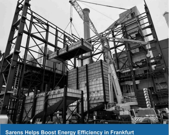
Sarens contributed to a significant project aiming at enhancing energy efficiency in Frankfurt, Germany. This project involved the installation of two horizontal HRSG
